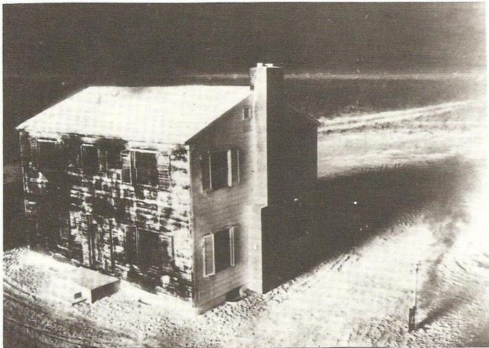
Figure 7.28b. Thermal effects on wood-frame house about 3/4 second later.
