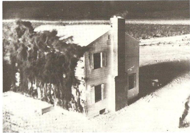
Figure 7.28a. Thermal effects on wood-frame house 1 second after explosion (about 25 cal/cm<sup>2</sup>).
