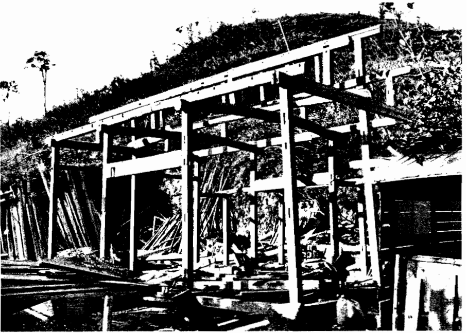
Figure 5.52. Upper photo; Wood-frame building; 1.0 mile from ground zero at Hiroshima. Lower photo: Frame of residence under construction, showing small tenons.
