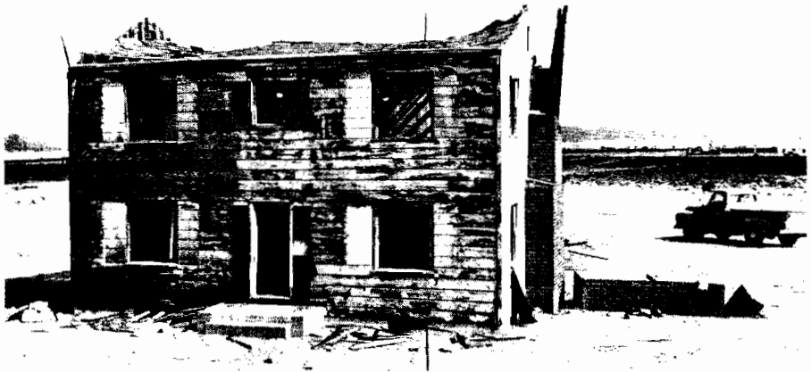
Figure 5.64. Strengthened wood-frame house after a nuclear explosion (4 psi peak overpressure).
